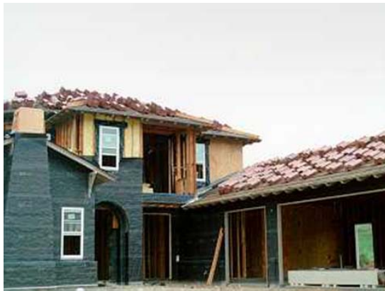
Phase 2 – roof loaded
