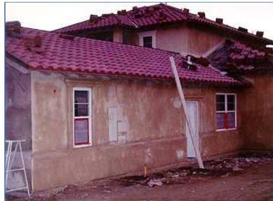
Phase 1 – roof with “hold-back”
