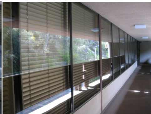
Second floor fenestration system
