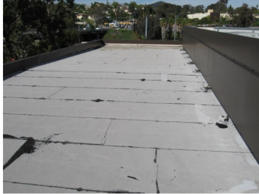
Flat Built-Up Roof
