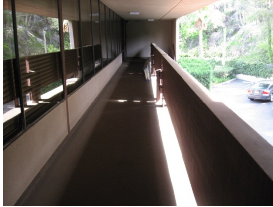
Second floor south elevation walkway
