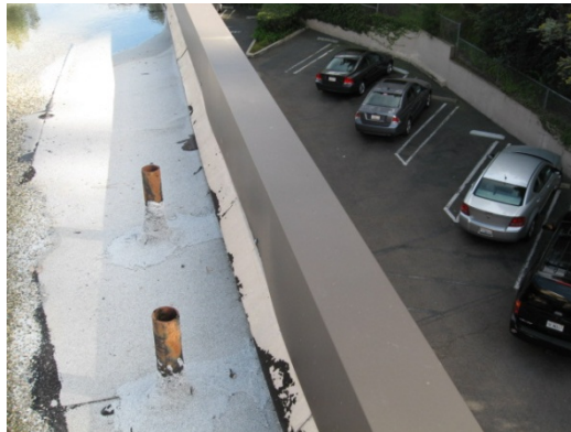
Sheet metal parapet cap.
